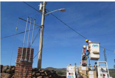
Cambio a Luminarias LED
